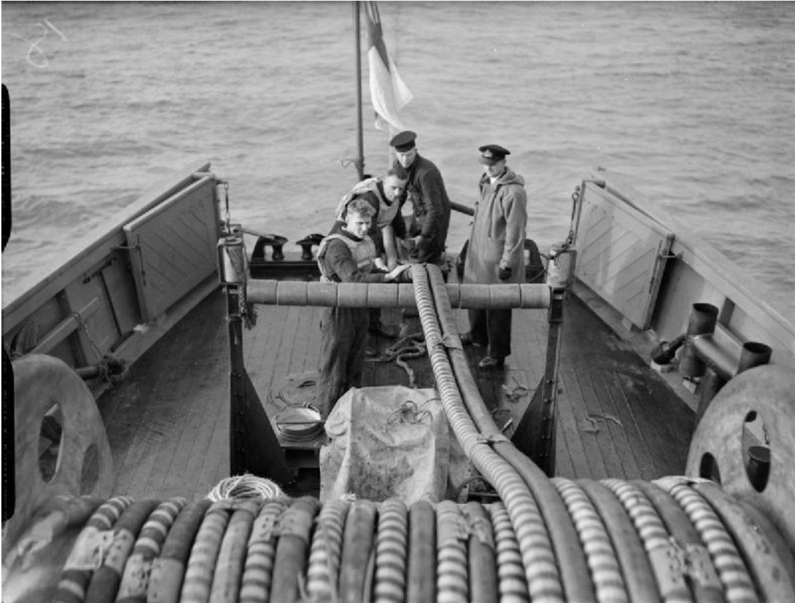
Figure 72 Archive image of buoyant electric minesweeping cable in use ©unknown
